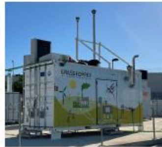
Figure 1. Grasshopper Pilot Plant in Abengoa's facilities
